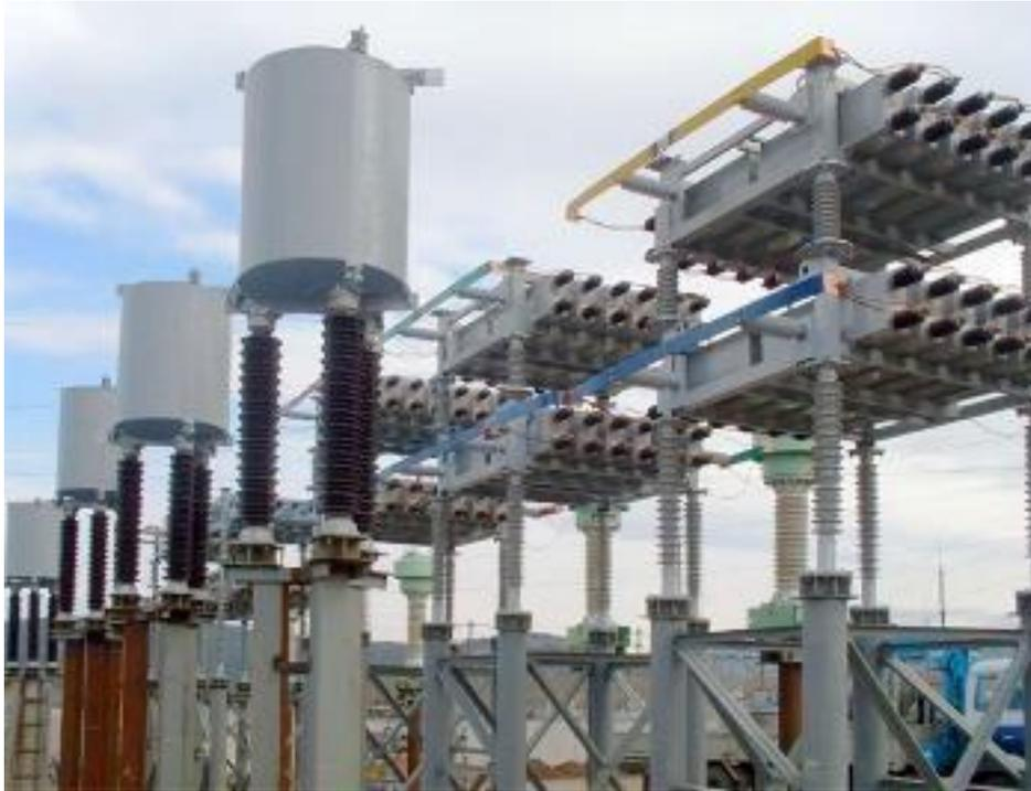
***Figure 4– Longitudinal compensation device at the substation***
